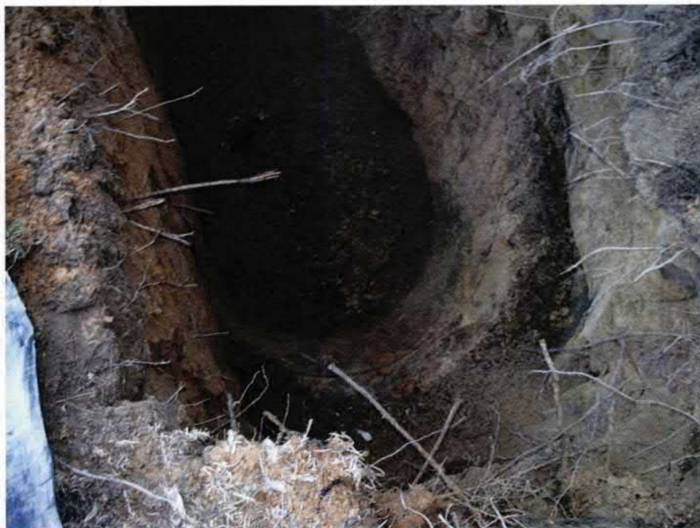
Picture 2: UST 702Bluebell tank pit.
